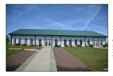
Known as the "Community Building", this 60' x 100' steel frame building with Big Ass fans has a concrete floor, an insulated metal roof, and metal and canvas siding. It has been used for large events and receptions. Adjacent to this building is a 25' x 40' frame restroom building.
