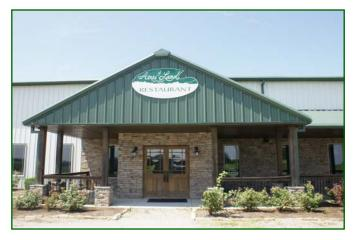
The restaurant is a 50' x 100' steel frame building with concrete foundation, metal and rock siding, and metal roof. It consists of hardwood flooring, two large walk-in coolers (7.75' x 15.75'), his and her restrooms with tile floors and walls, plus a wrap-around porch. There is natural gas heat and central airconditioning plus a generator.
