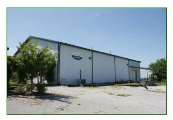
The winery is a 60' x 100' steel frame building with metal siding and roof. It consists of concrete floors, overhead doors, and is partitioned. There is a 14' x 24' loading dock, and the building has natural gas heat and central airconditioning.
