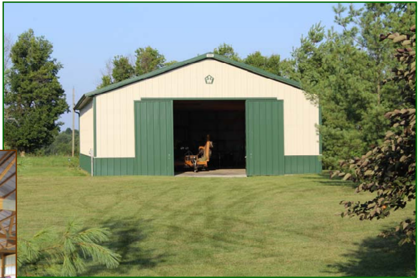
36' x 64' Walter storage building with concrete floor and insulated roof.
