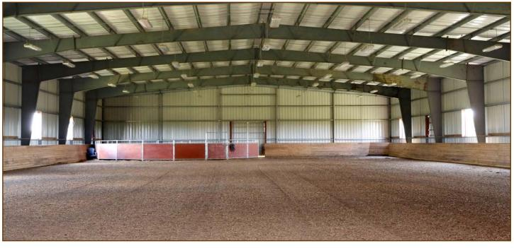
State-of-the-art 100' x 240' steel building featuring a 30.48m x 60.96m indoor arena (riding area measures  $28.6m \times 59.74m$ ). The footing is cedar chips over a solid clay base then limestone sand and top soil. All 16 windows open which gives the feeling of a covered arena and provide for excellent ventilation. Containing 12 stalls, 2 wash bays, an 11' x 25' tack room with full bath and washer/dryer hookup.
